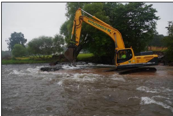
Figure 9. Removal of the weir
