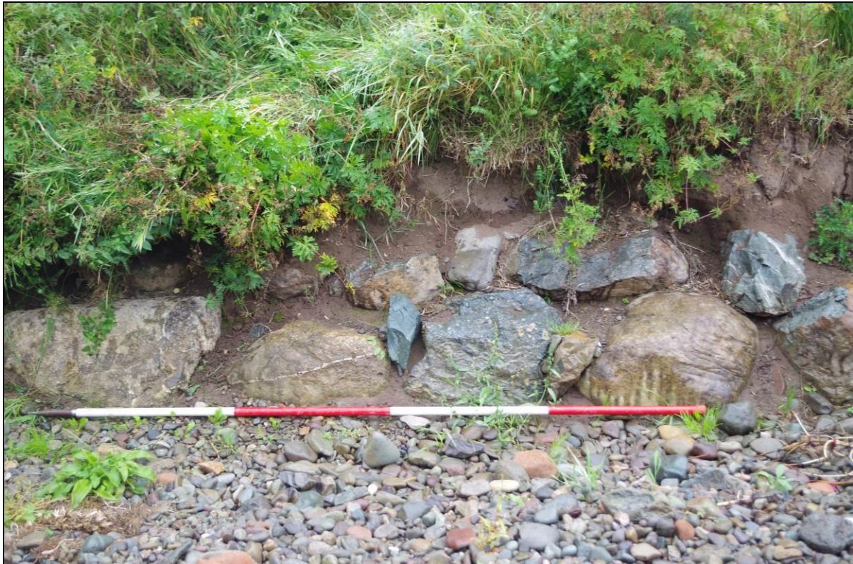
Figure 15. Stone revetment
