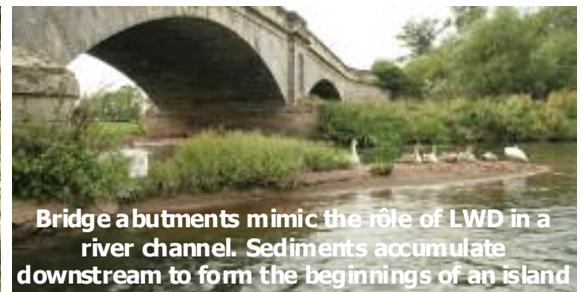
**Bridge abutments mimic the rôle of LWD in a river channel. Sediments accumulate downstream to form the beginnings of an island**
