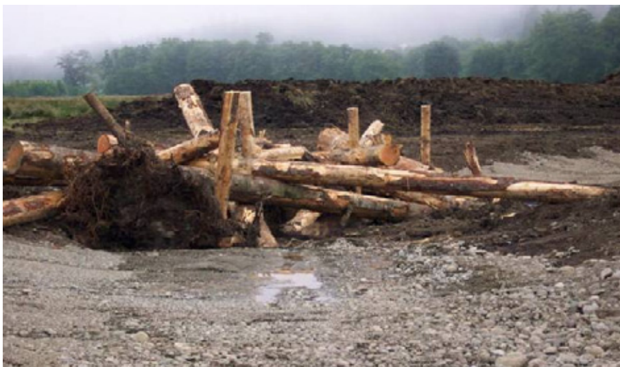
Plate 3 LWD dam using piling for stabilisation (Stream Habitat Restoration Guidelines (2004)).
