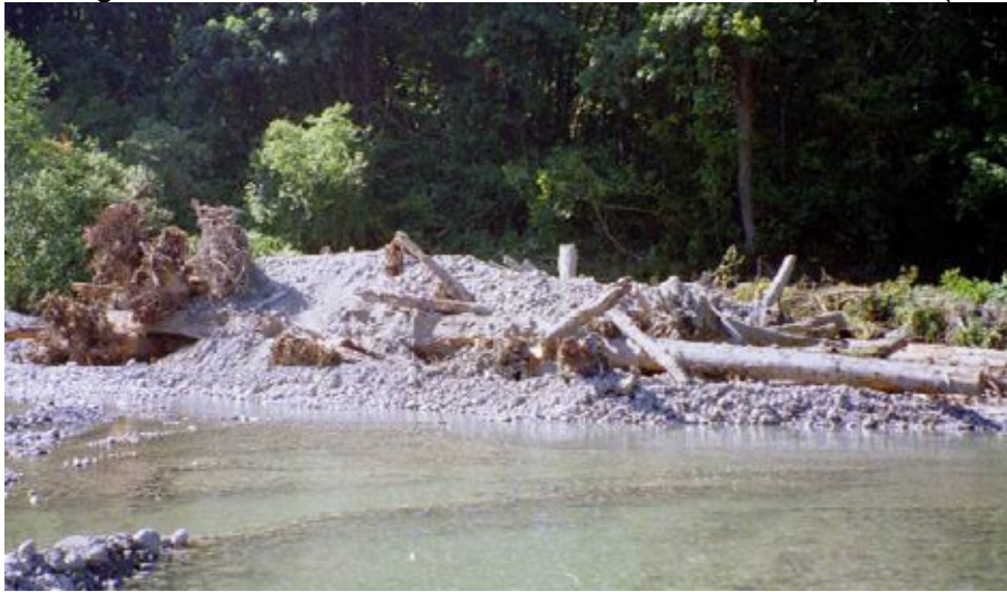
Plate 2 LWD dam anchored using ballast (Stream Habitat Restoration Guidelines (2004)).
