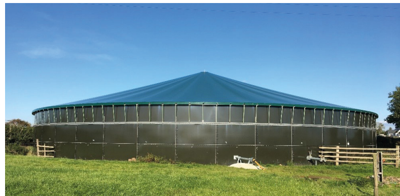
Covered slurry store.
