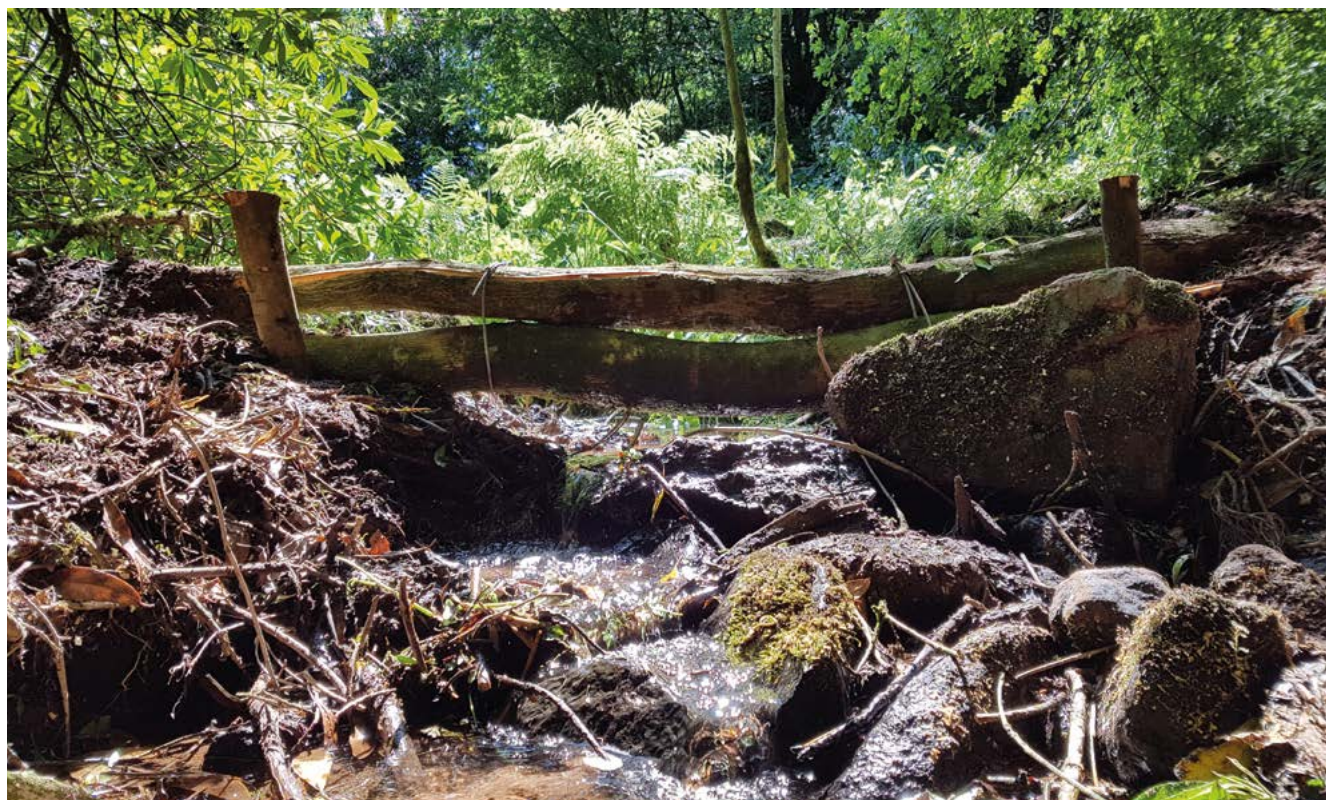
Leaky dams in Cumrew © ERT
