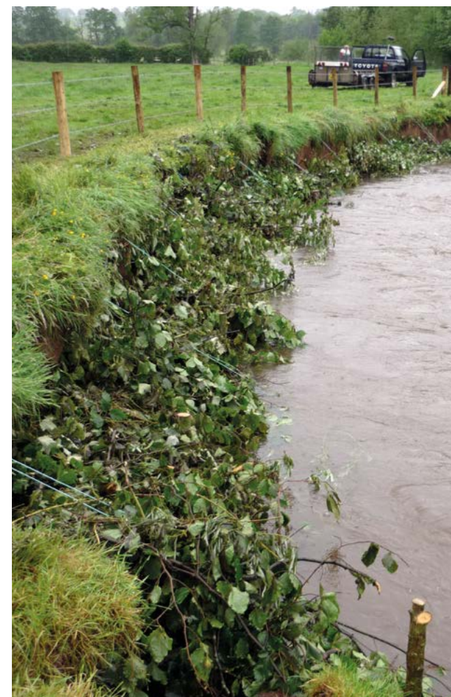
Large woody debris installed to protect the riverbank in the Petteril © ERT
