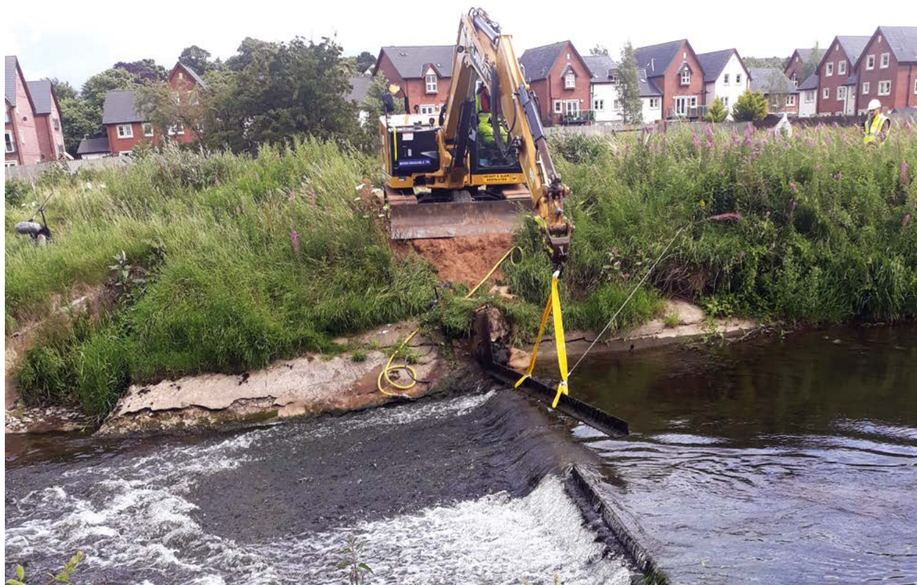
Removal of weir in Carlisle © ERT
