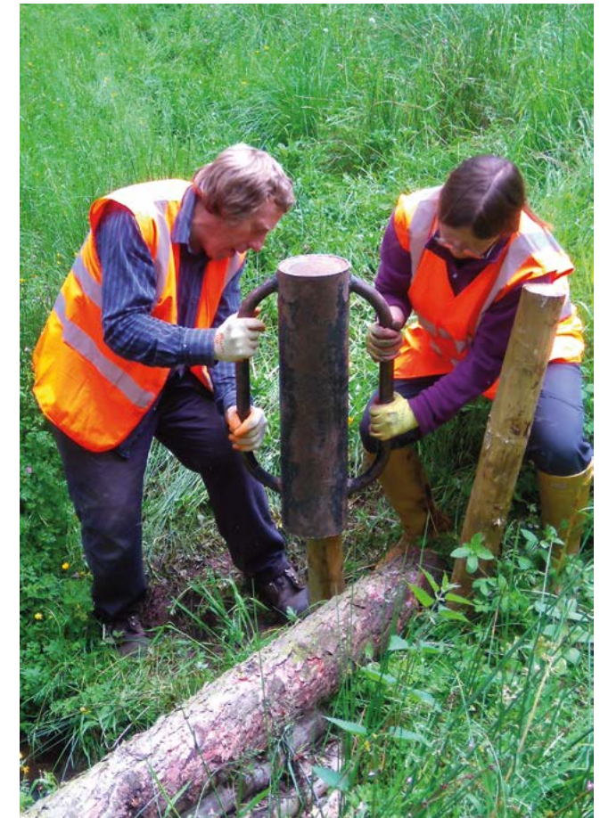
Volunteers building leaky dams © ERT
