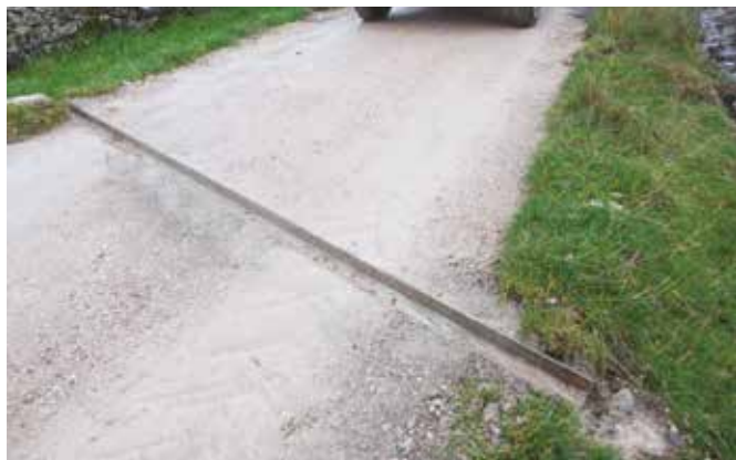
Cross drain to divert run-off from a farm track. © West Cumbria Rivers Trust.
